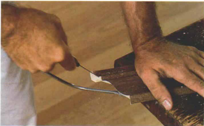
Before the crown molding can be coped, the end must be mitered to expose the profile. Positioned "upside down and backwards" in the miter box, the molding rests against small nails that hold it at the proper angle (top left). After exposing the profile of the crown molding, the back part of the stock is cut away with a coping saw, which must be held at a severe angle or the coped joint will not be tight (left). Even with the coping saw cutting at a severe angle, it's tough to remove enough wood through the S-curve in crown molding. Additional stock often has to be pared away with a utility knife (above).
