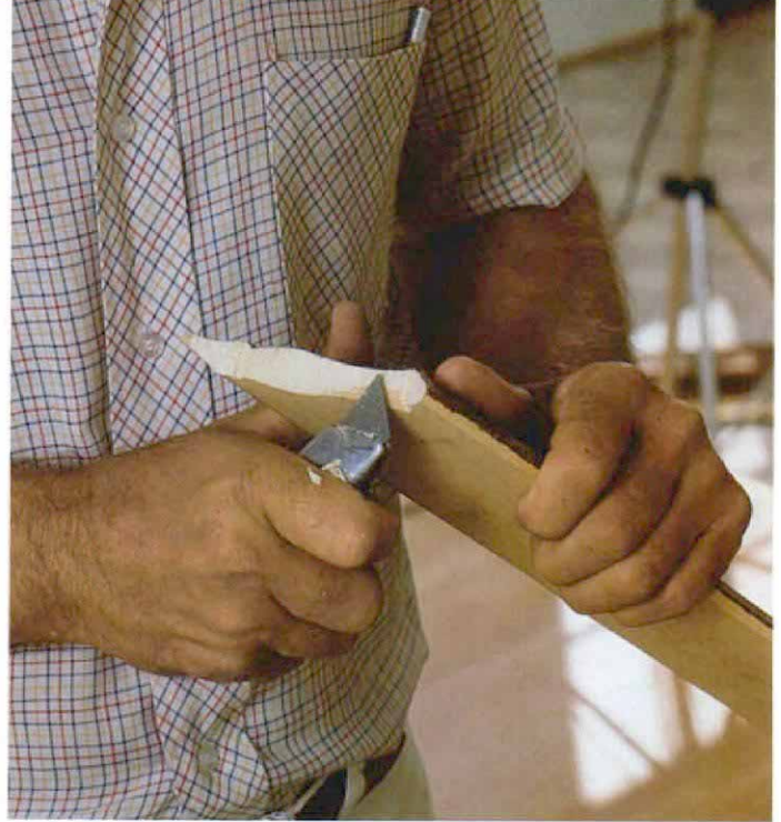
Before the crown molding can be coped, the end must be mitered to expose the profile. Positioned "upside down and backwards" in the miter box, the molding rests against small nails that hold it at the proper angle (top left). After exposing the profile of the crown molding, the back part of the stock is cut away with a coping saw, which must be held at a severe angle or the coped joint will not be tight (left). Even with the coping saw cutting at a severe angle, it's tough to remove enough wood through the S-curve in crown molding. Additional stock often has to be pared away with a utility knife (above).
